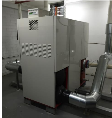
Multistack MagLev oil-free modular chiller
