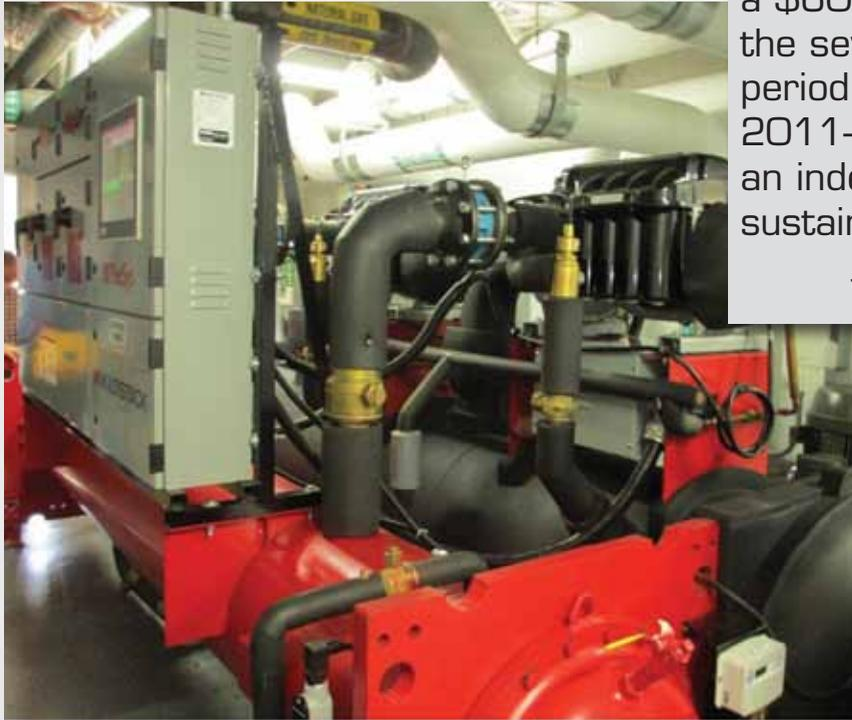
*The 300-ton Multistack chiller at Windy Hill Hospital uses MagLev™ compressors for optimum efficiency and reliability while virtually eliminating compressor maintenance needs.*
